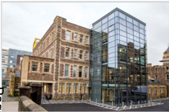
New One Stop Shop in Cardiff
